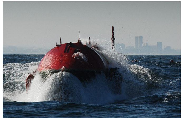
Fig. 6. The front of the Pelamis machine bursting through a wave at the Agucadoura Wave Park of Portugal. [33]
